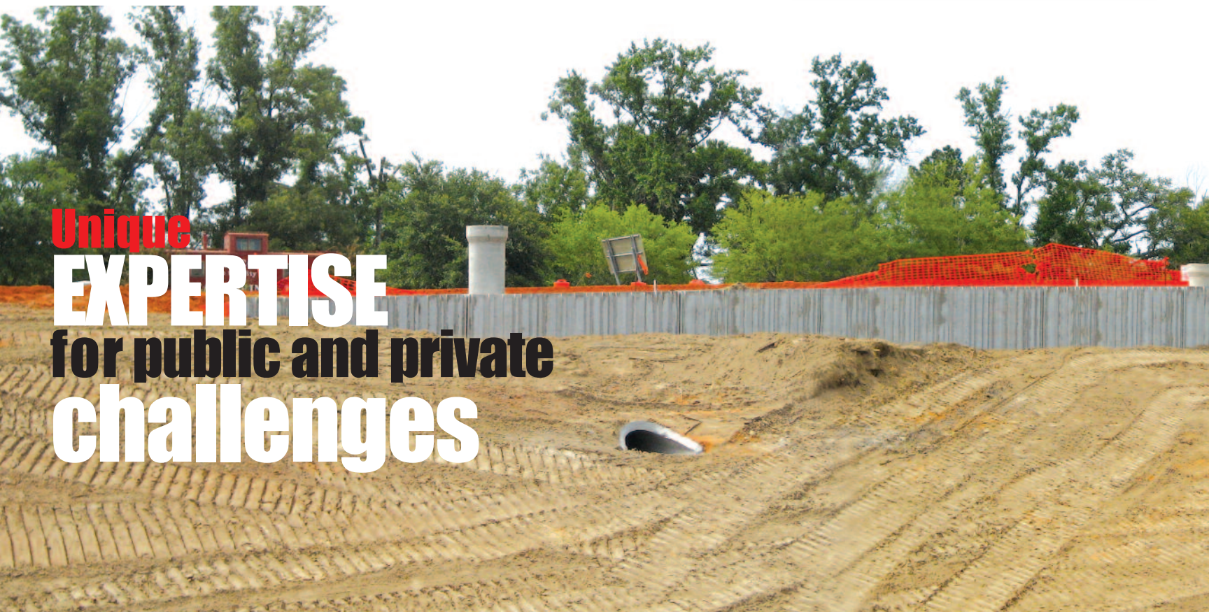
Mississippi Department of Transportation - Biloxi, MS and Pass Christian, MS 17,000 s.f. and 3,000 s.f. 2-stage MSE retaining wall bridge lead up ramps with full-height precast concrete panels. (Two of the many bridge structures rebuilt after Hurricane Katrina.)
