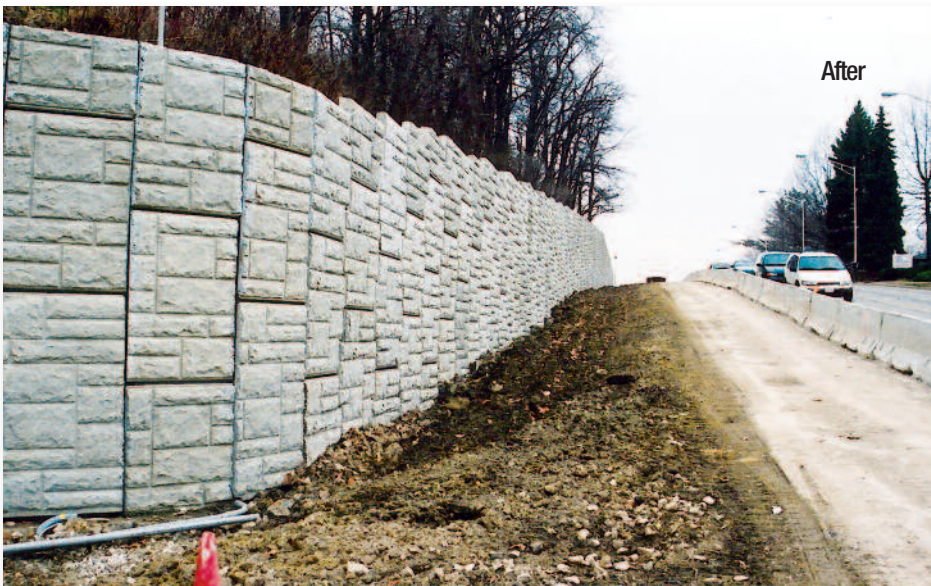
Sam's Club - Cuyahoga Falls, Ohio 8,000 s.f. rock anchor assisted precast concrete panel MSE retaining wall
