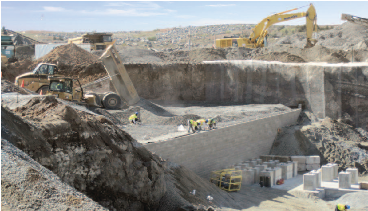
Dolese Bros. Aggregates Mine and Manufacturing facility - Roosevelt, OK 5,000 s.f. segmental block MSE retaining wall dump structure, 38' tall Simultaneous installation; dump structure and primary crusher
