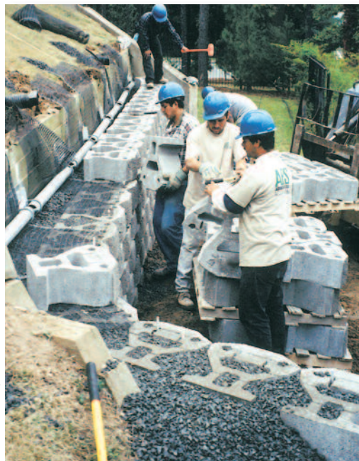
Replacement of failing timber wall with soil nails and a segmental block facing - Little Rock, AR
