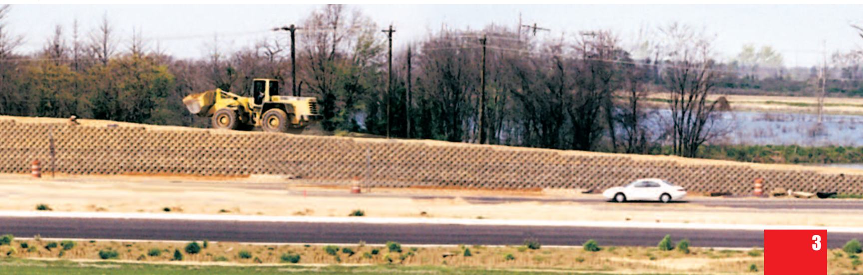
Mississippi Department of Transportation - Yazoo City, MS 13,200 s.f. segmental block MSE retaining wall bridge lead up ramps
