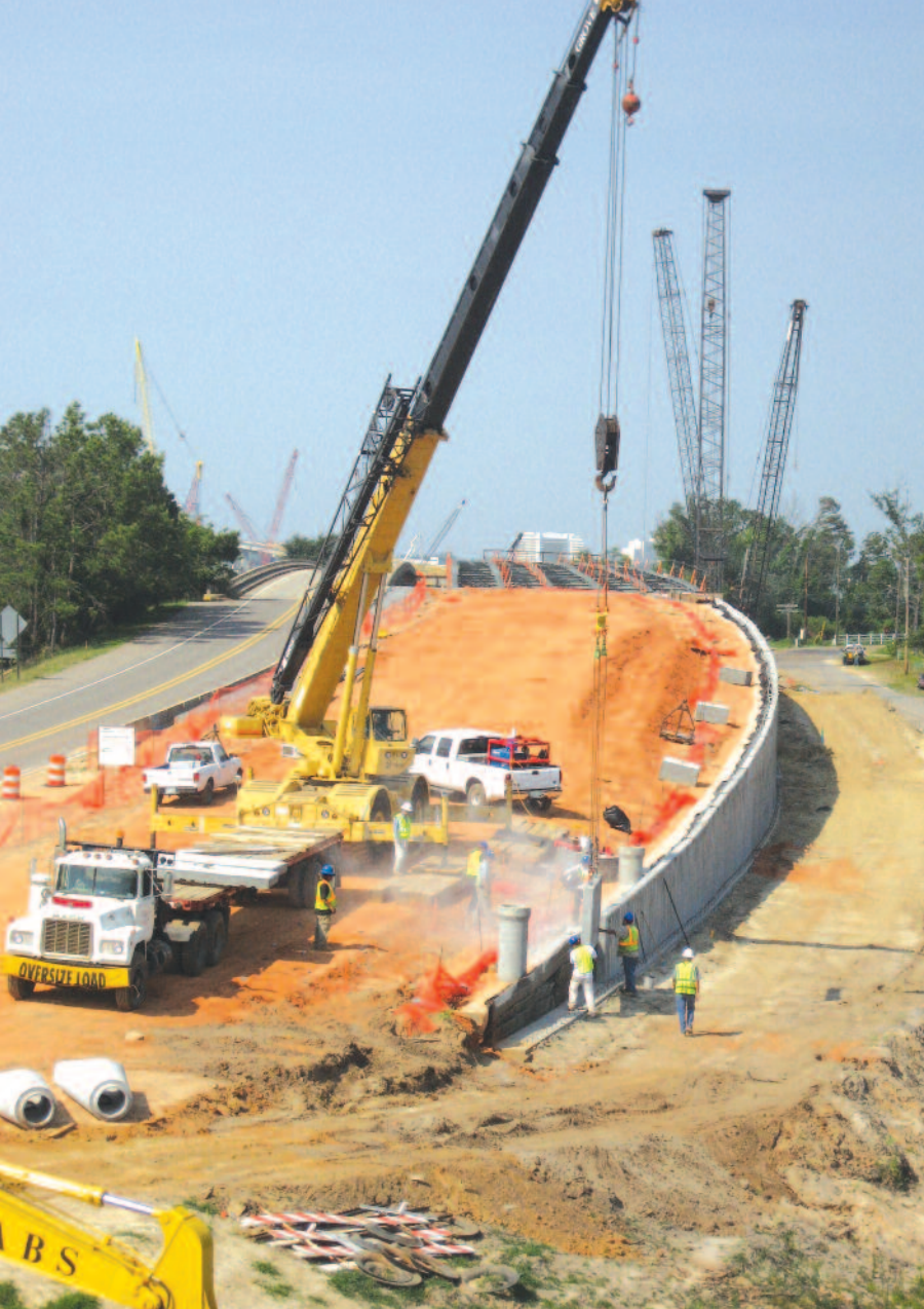
Mississippi Department of Transportation - Biloxi, MS and Pass Christian, MS 17,000 s.f. and 3,000 s.f. 2-stage MSE retaining wall bridge lead up ramps with full-height precast concrete panels. (Two of the many bridge structures rebuilt after Hurricane Katrina.)
