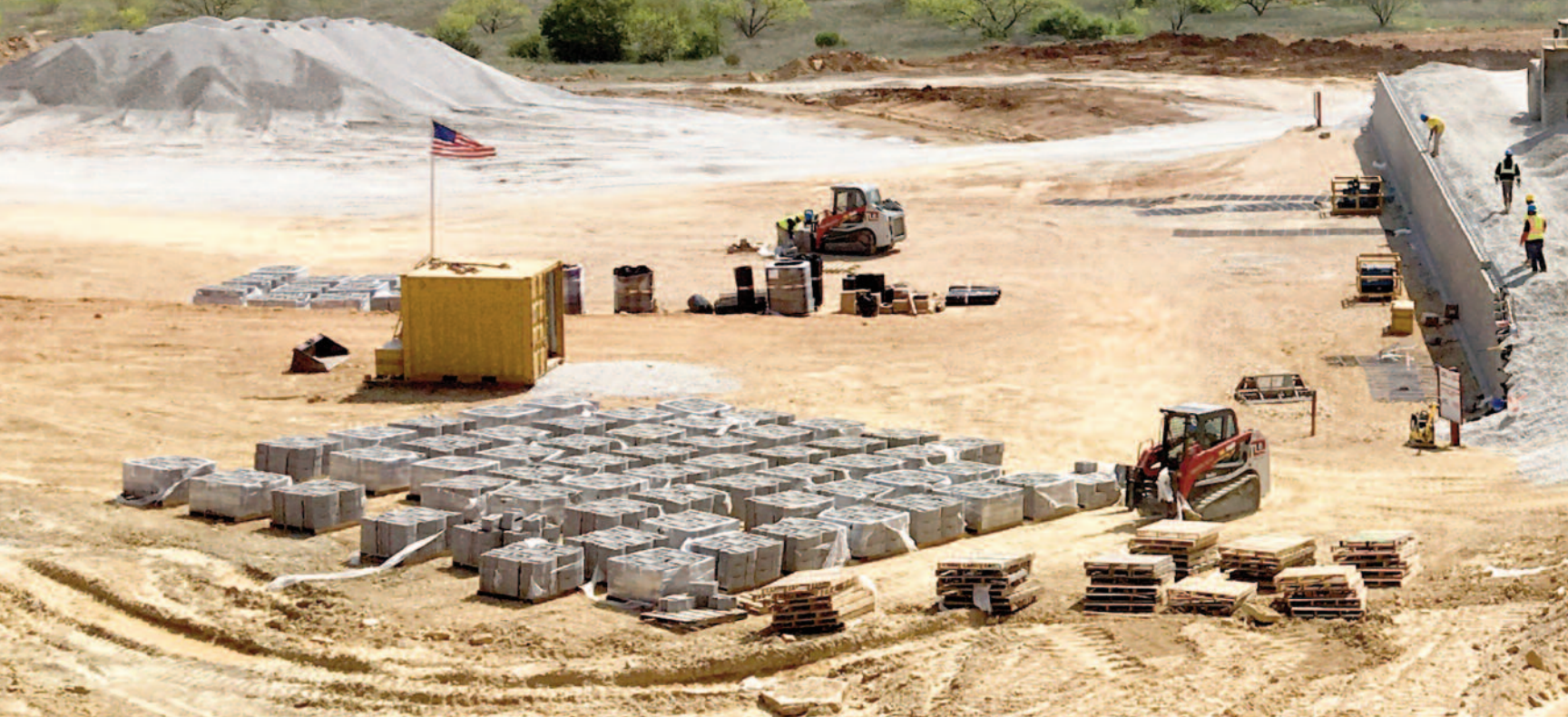
Aggregates Mine Millsap, Texas 8,000 s.f. segmental block MSE retaining wall dump structure and lead up ramp, 43' Tall
