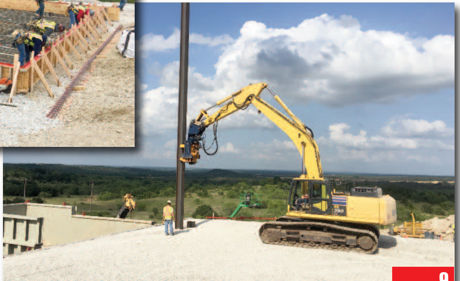
Steel H-piles installed with 100 ton high-frequency vibro hammer
