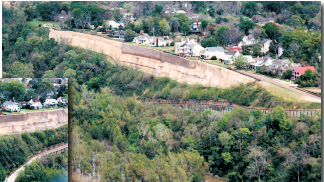
Natchez Bluff Slope Stabilization - Natchez, MS 70,000 s.f. multi-strand soil anchor and soil nail wall with permanent shotcrete facing and 18,000 s.f. MSE retaining wall.
