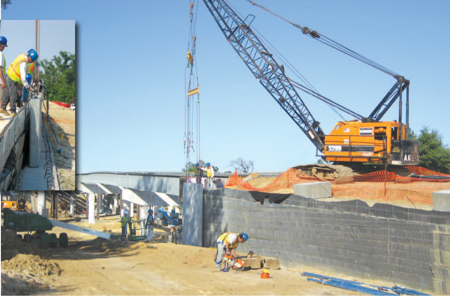
2-stage welded wire MSE retaining wall with full-height precast concrete panels.
